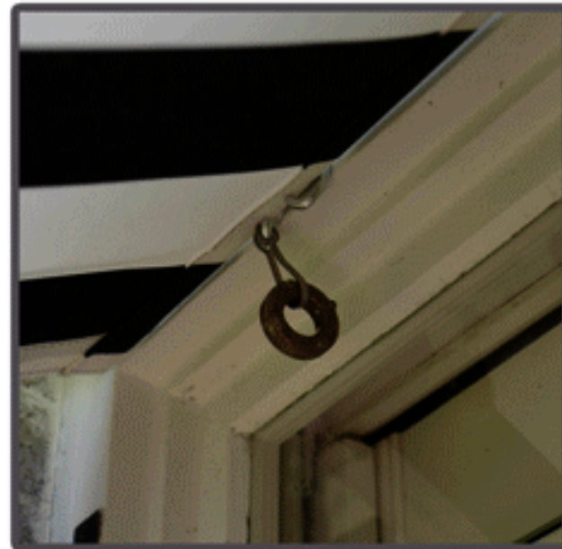
Slip ring pulley over hook on headrod clamp.
