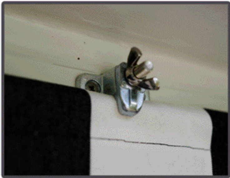
Headrod Clamp- Clamp over fabric and tighten wingnut.
